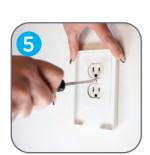
Place Mounting Plate and Insert over the outlet with the Qdos logo at the bottom and secure firmly with provided screws.
