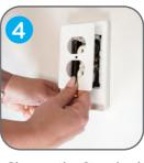
Choose the Standard or Decora Insert depending on your Wall Plate style, and fit Insert into the Mounting Plate
